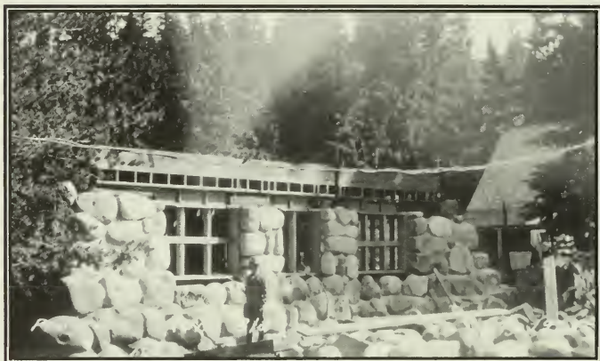
During excavation all big boulders were saved and used by the stone mason. The structure, 37 feet by 64 feet, has boulder walls to the second story windows with Alaska Cedar slab construction above, July 1928. (Park Structures Collection)
